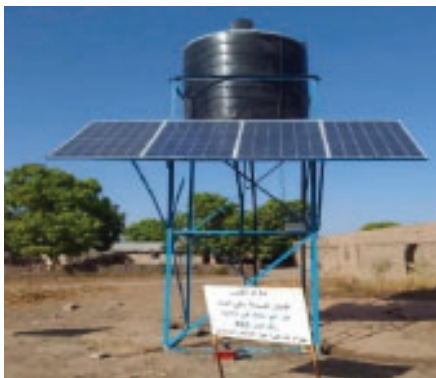
The first picture (left) shows the complete installation of Borehole upgraded with solar powered water pumping, and improved storage, the second image (right) a briefing of water committee members who have caretaker roles to manage and maintain the boreholes.
